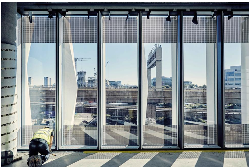
The building is adjacent to the Westway. The fins provide protection from headlight glare at night from cars
